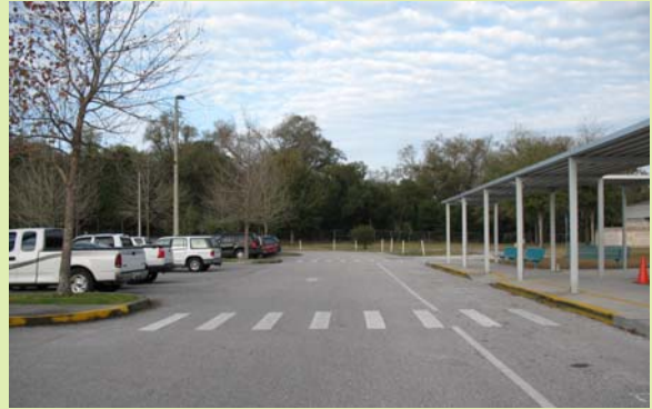
The crosswalk does not align with curb ramps
